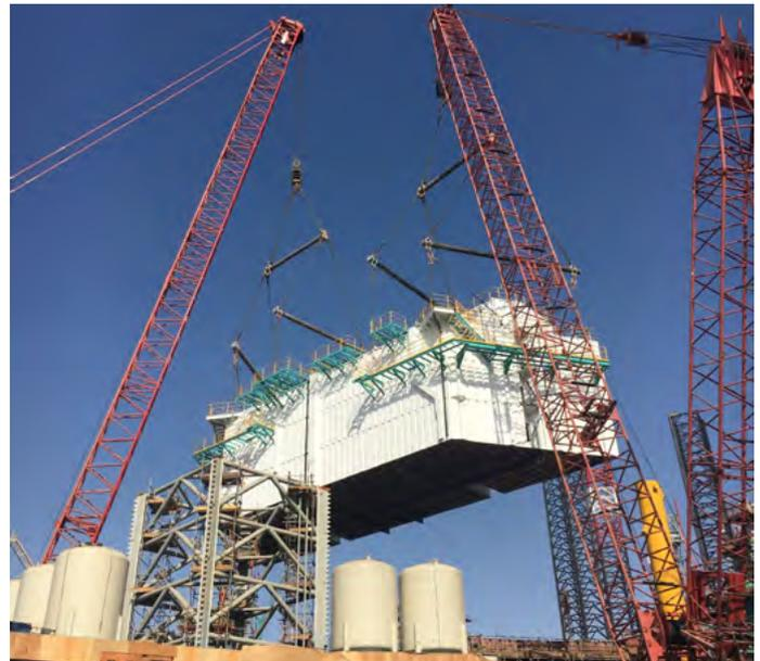
In May the NDC 8 accommodation module was lifted on board the rig and installed successfully
