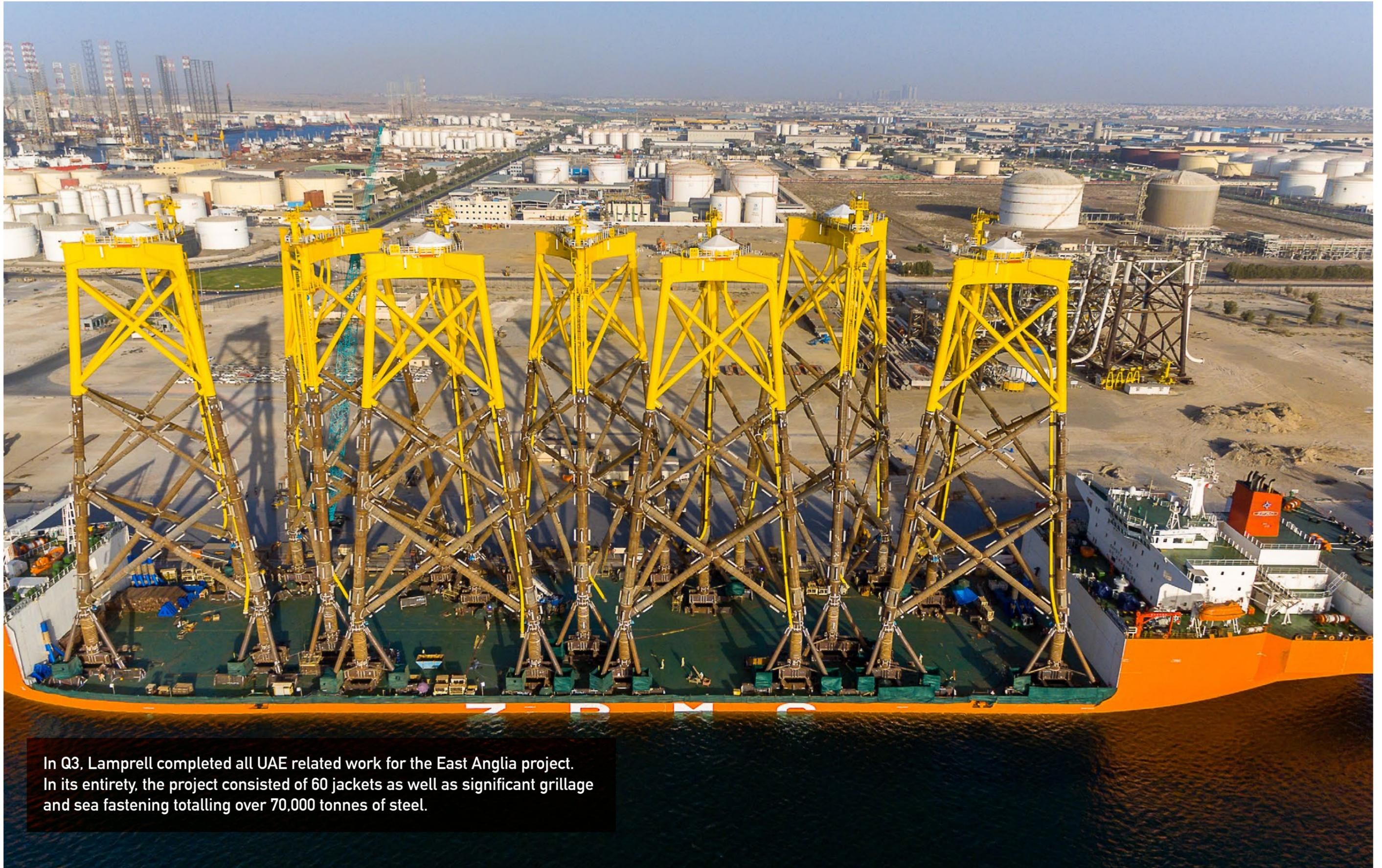
In Q3, Lamprell completed all UAE related work for the East Anglia project. In its entirety, the project consisted of 60 jackets as well as significant grillage and sea fastening totalling over 70,000 tonnes of steel.
